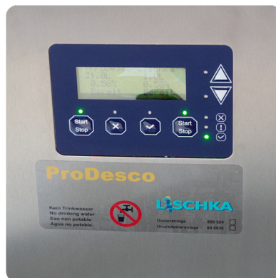
Mixing unit for cleaning solution fitted in the base cabinet
