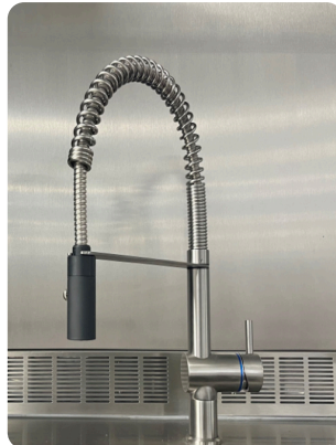
Cleaning spray head for hot water/cold water mounted under the protective hood
